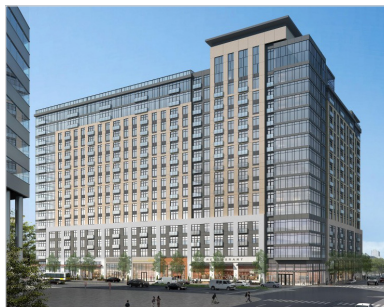
The Smyth - 885 Washington Blvd 414 apartments & 19,000 sf retail Estimated Completion: 2022
