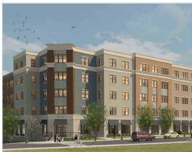
Park 215- 215 Stillwater Ave 78 Units & 24,000 sf commercial Estimated Completion: Q3 2018
