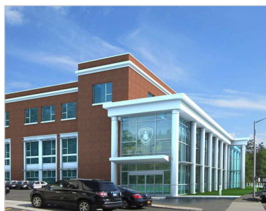
Stamford Police Station- 805 Bedford St 94,000 sf Police Station Estimated Completion: Q1 2019
