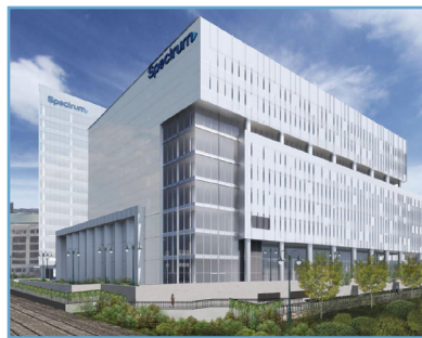
Charter Communications World HQ 777,000 sf commercial Estimated Completion: 2020
