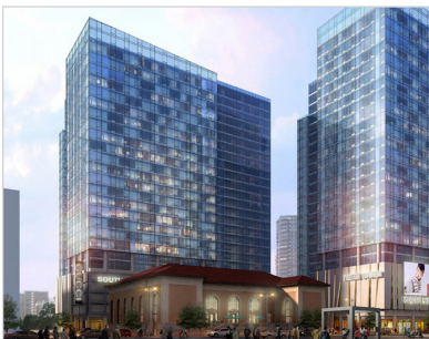
Atlantic Station Phase 2 - 421 Atlantic St 323 units & 14,000 sf retail Estimated Completion: Q2 2021
