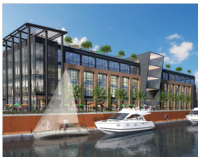
ITV America HQ- 860 Canal St 130,000 sf commercial Estimated Completion: 2021
