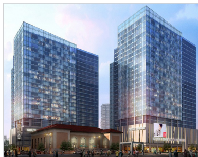
Atlantic Station Phase 2 - 421 Atlantic St 325 units & 14,100 sf retail Estimated Completion: Q2 2021
