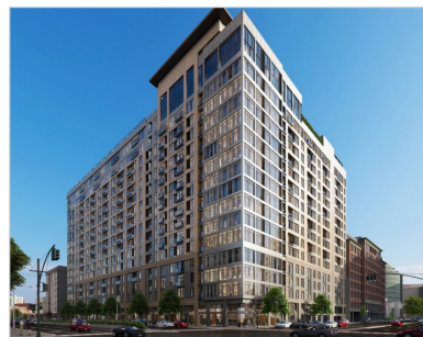
The Smyth- 885 Washington Blvd 414 units & 19,333 sf retail Estimated Completion: Q3 2021
